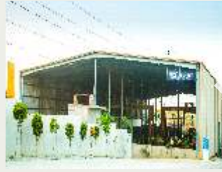
BCC PRECAST PLANT
